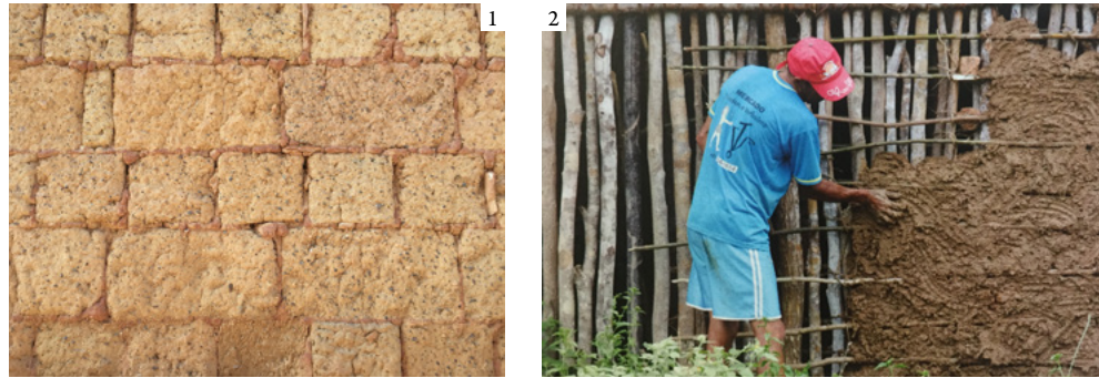
1: Adobe wall in Goiás, 2019 2: Taipa de enchimento in the village of Iuna, Lençóis, state of Bahia (Lins and Santana 2017: 21)
