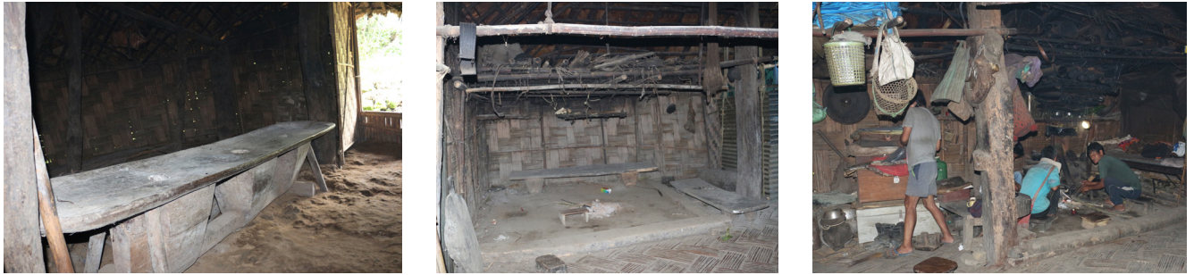
Figure 8. Tham rice pounding tool and fire place. The smoke of the latter disinfects the interior of the house and forms a soot layer over the bamboo in a way that protects the bamboo from insects and corrosion
