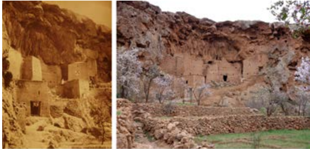
Granary of Ifri Imadiden, Sirwa, in 1948 (D. Jacques-Meunié), and before and during its restoration in 2018-19 (D. Goeury)
