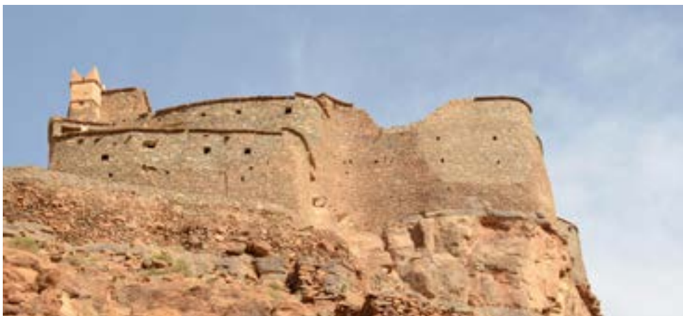
Agadir n'Uguellouy, Western Anti-Atlas, before and after the restoration of 2016
