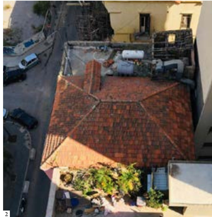
1: Damaged roof tiles 2: Tile replacement (1,2: Youssef Kassar)
