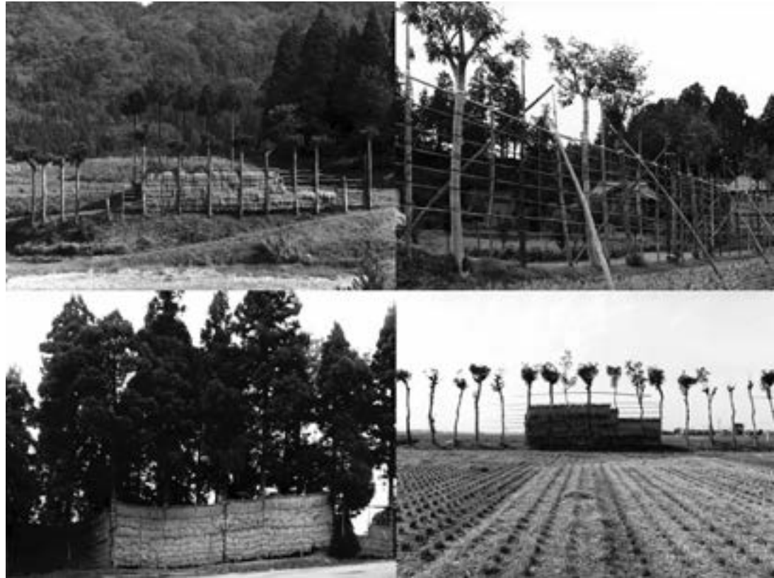
Figure 21a. These makeshift structures are erected in hours. They need scarcely any maintenance. They consume no material apart from rope. Once dismantled, the place is left as it was before. Economy and ecology at their best! (Sanpoku machi-Ogoto)
