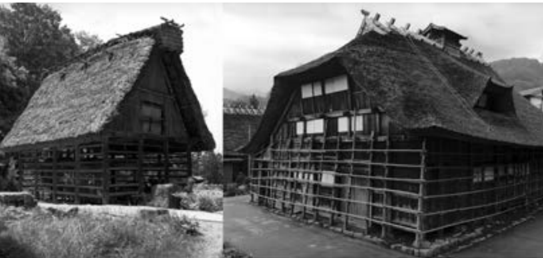
Figure 20a. This double cereal drying rack with storage space under the roof makes use of the open gable for extra hanging capacity (Shirakawa-mura)
