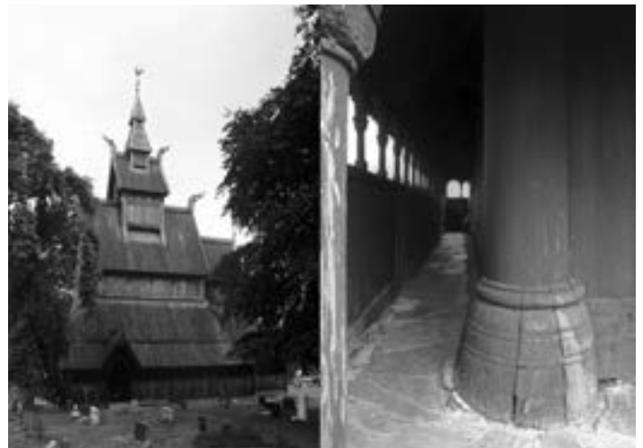
Figure 9b. Corner pillar of the church in Hopperstad
