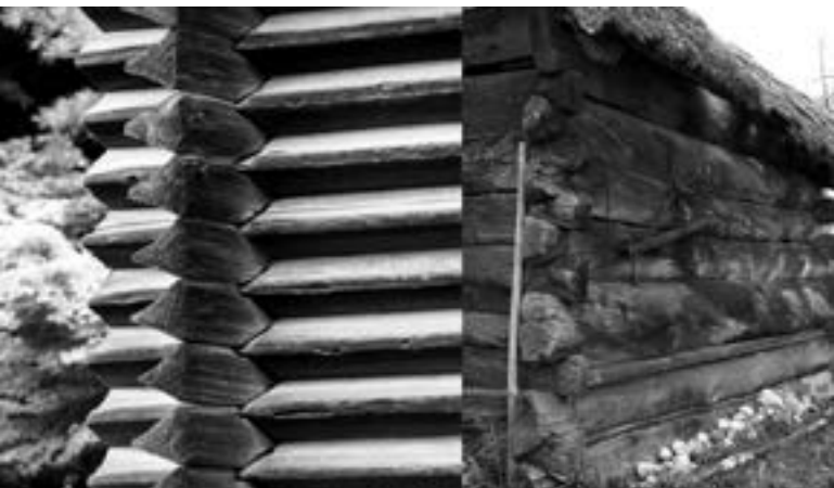
Figure 15a. Detail of a corner of Tōshōdai-ji hozo in Nara Figure 15b. This log building in Kruszyniany, Poland, is built of halved logs. The advantage of flat inside walls cannot offset the building's poor execution
