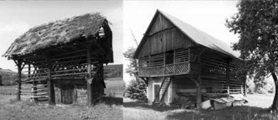
Figure 19a. Drying ladders can be hung around house walls (Matting, Austria)
