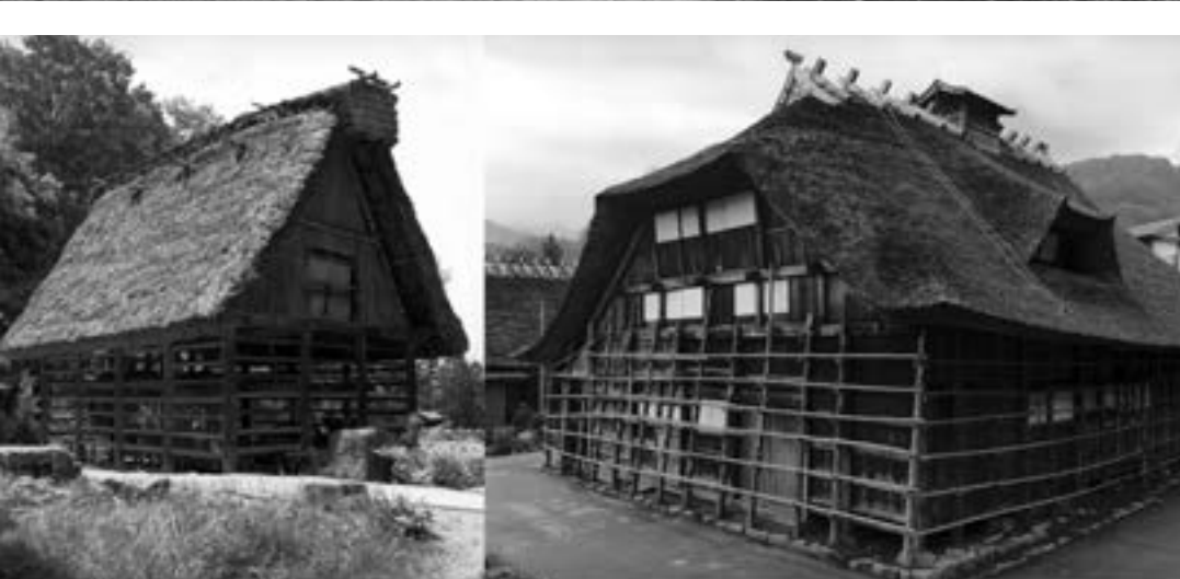
Figure 20a. This double cereal drying rack with storage space under the roof makes use of the open gable for extra hanging capacity (Shirakawa-mura)
