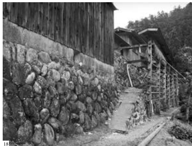
Figure 17. Single drying racks need braces against the wind, and these have to be installed in a way that does not make the rack difficult to handle (Abfaltersbach, Austria)
