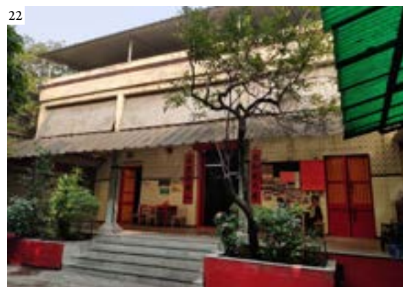
Figure 22: View of the Nam Soon Temple from its front yard
