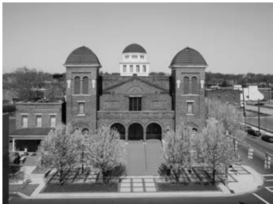
Figure 4: 16th Street Baptist Church by Wallace A. Rayfield, Birmingham, Alabama, 1911 (Library of Congress)
