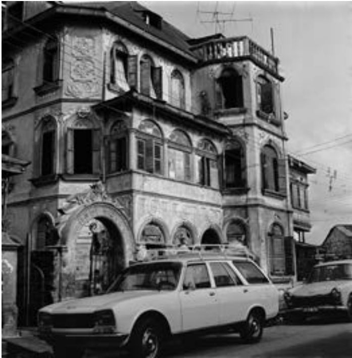
Figure 13: Ēbùn House by Sàró architect Herbert Macaulay and Afro-Brazilian craftsman Balthazar dos Reis, Lagos, Nigeria, 1913 (Salvador, Brazil: Fundação Pierre Verger)
