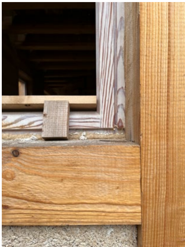
Window detail from outside and from inside | Detalle de la ventana desde el exterior y el interior | Pormenor da janela vista do exterior e do interior
