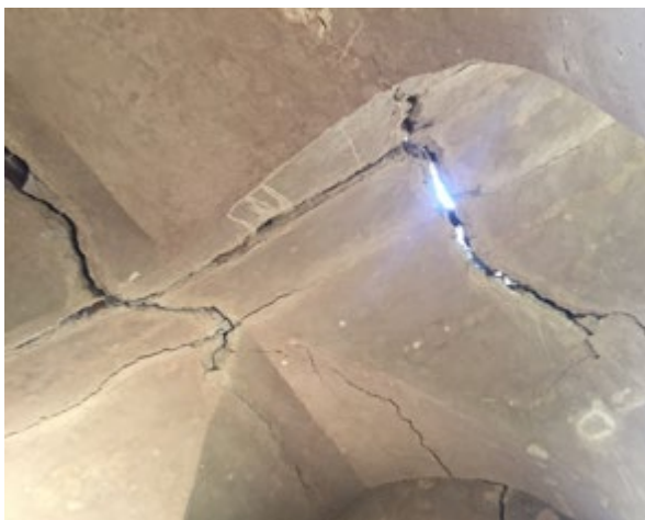
Figure 8: Cracked ceilings | Techos agrietados | Tetos com fissuras
