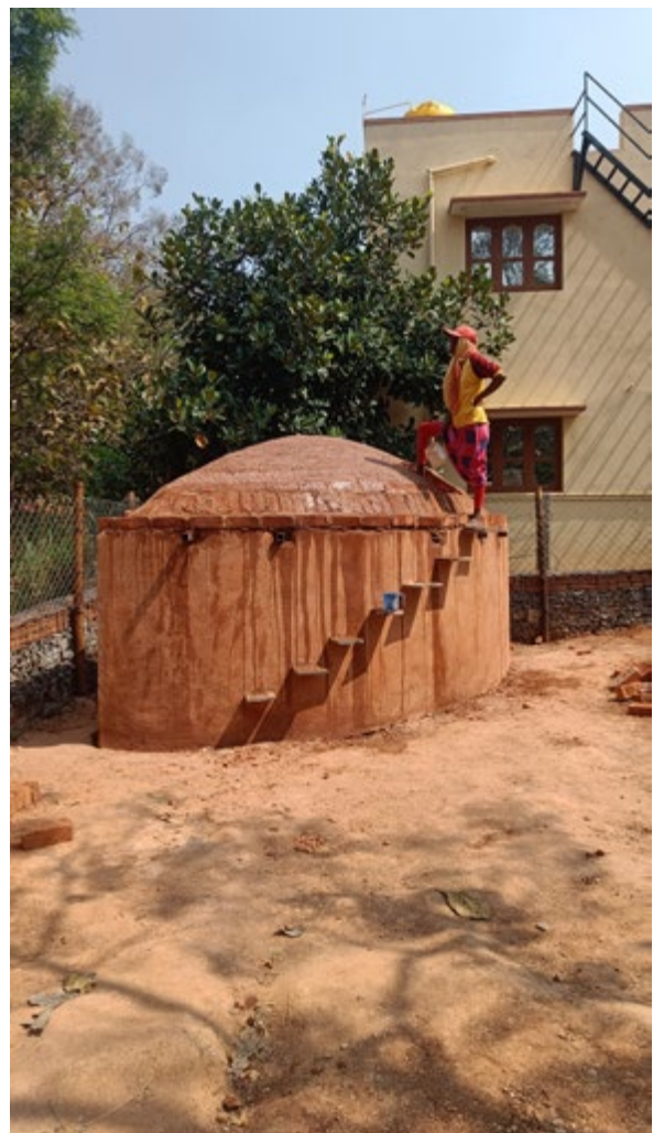
Figure 4: Thappi plastering on a brick and lime mortar water tank (Bagalur, India, 2023)
