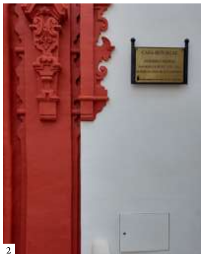
1, 2: Details of the brick-cut and carved doorway 3: Main façade with a double-bay “altarpiece-style” doorway and a three-arched tower seen from San Sebastián Street | 1, 2: Detalles de la portada de ladrillo cortado y tallado 3: Fachada principal con portada de doble tiro (“tipo retablo”) y torreón de tres arcos desde la calle San Sebastián | 1, 2: Detalhes do portal em tijolo cortado e esculpido 3: Fachada principal com portal de duplo vão (“tipo retábulo”) e torre de três arcos vista da rua San Sebastián (1, 2: Alejandro García Hermida 3: Fernando Alda)
